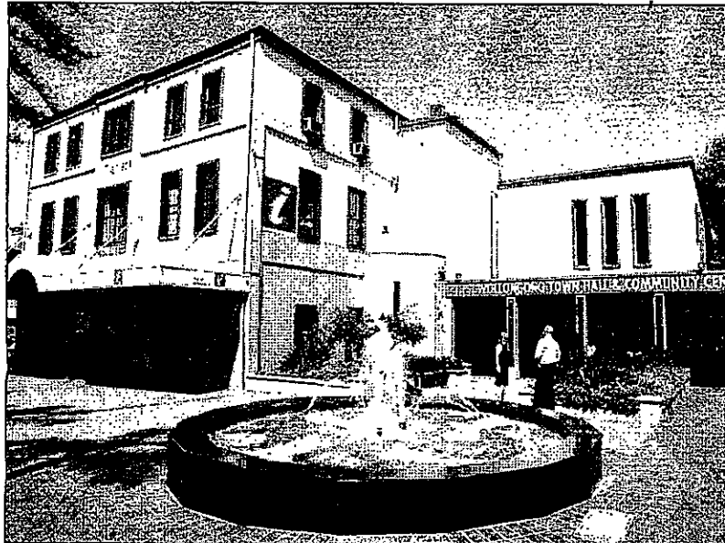
The first stage of renovation works to the Wollongong Town Hall will commence with the removal of lead dust and asbestos.
