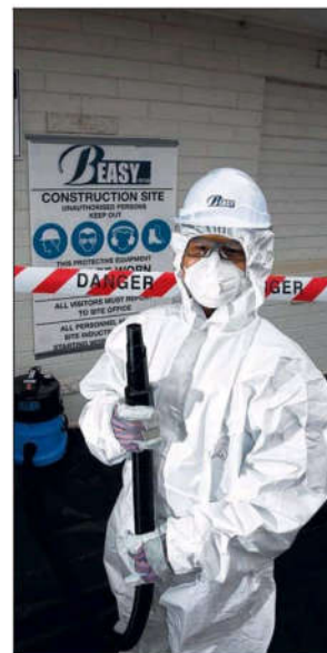
Asbestos removalist Bret Baker in protection gear. Picture: ROBERT POZO
